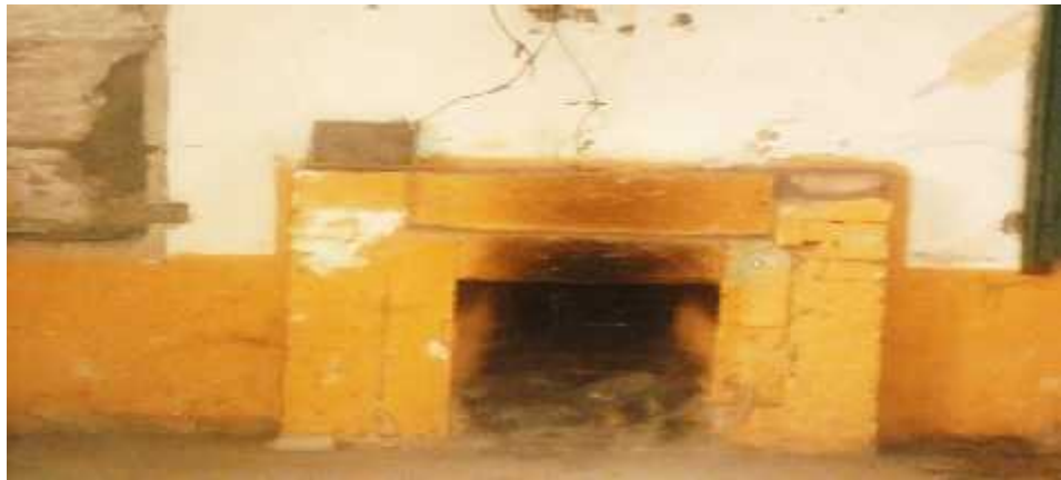
Figure 10 - Chimney on the second floor
